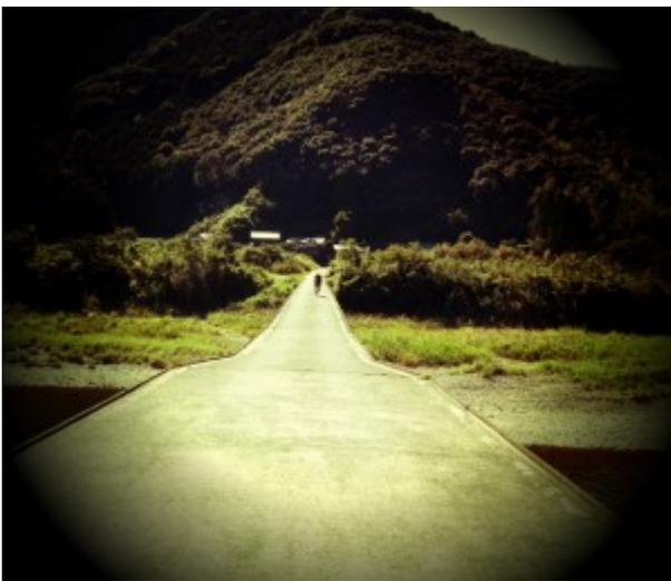
10. After the shows were over Peet and I went for a ride. This is Peet riding across a Chinkabashi, which is a specially designed bridge intended to sink peacefully and steadfastly in the event of flood (hence, no railing). The Shimanto River in Shikoku is one of the last clear water rivers in Japan and was stunning to ride along, though our ride was cut short by the onset of a typhoon.
